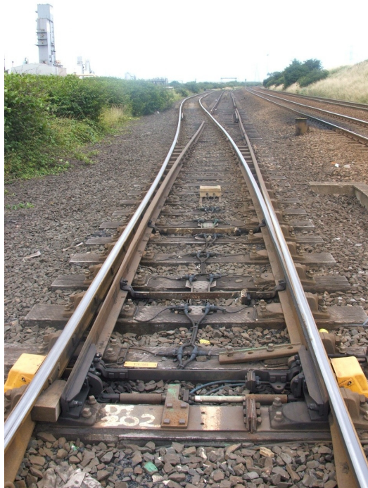
Figure 18.2 Shell Junction looking in down direction
