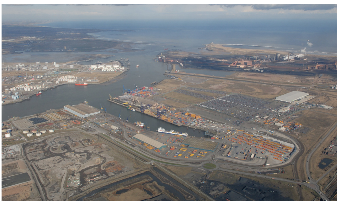
Figure 21.1 Photograph showing the industrialised nature of the lower Tees estuary, looking seawards
